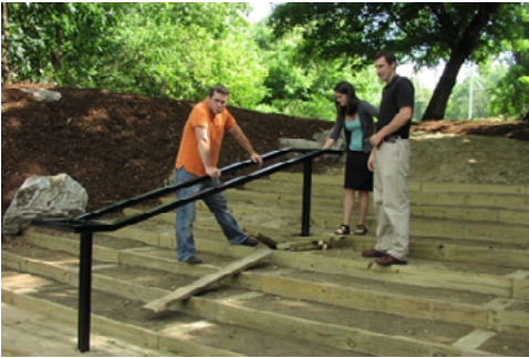
Figure 15 Wooden Stairs Source: sds-la.com
