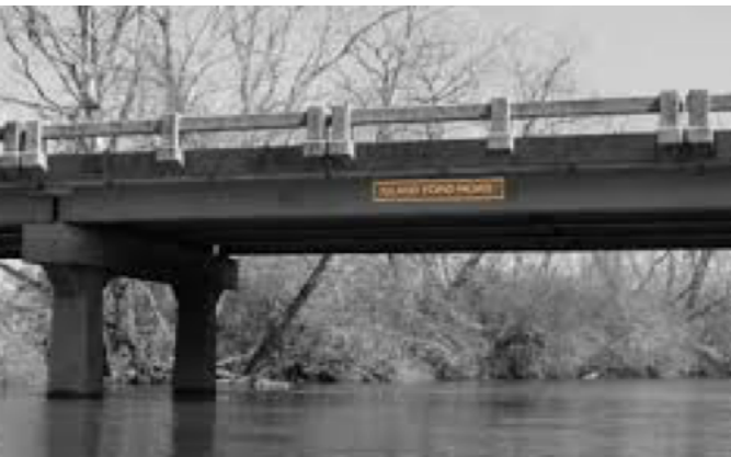
Figure 22 Example Bridge Signage Source: americantrails.org
